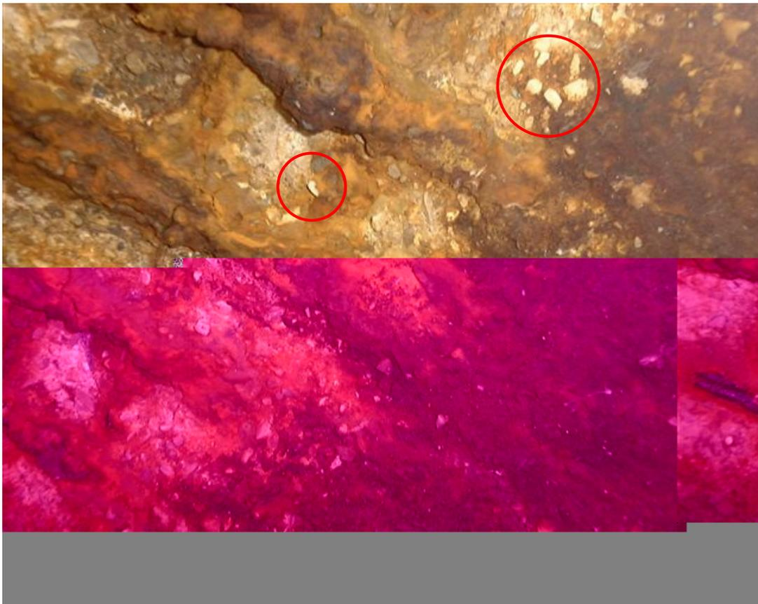
Figure 1. Close-up of a 900 mm concrete sewer pipes that experienced severe MIC. The steel reinforcement ribs are either gone or in an advanced corrosion state. The white solids are MIC corrosion products (marked by red circles)
